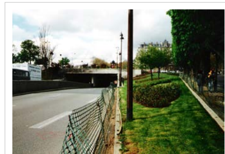
East entrance to the Pont de l'Alma tunnel in Paris [21]
